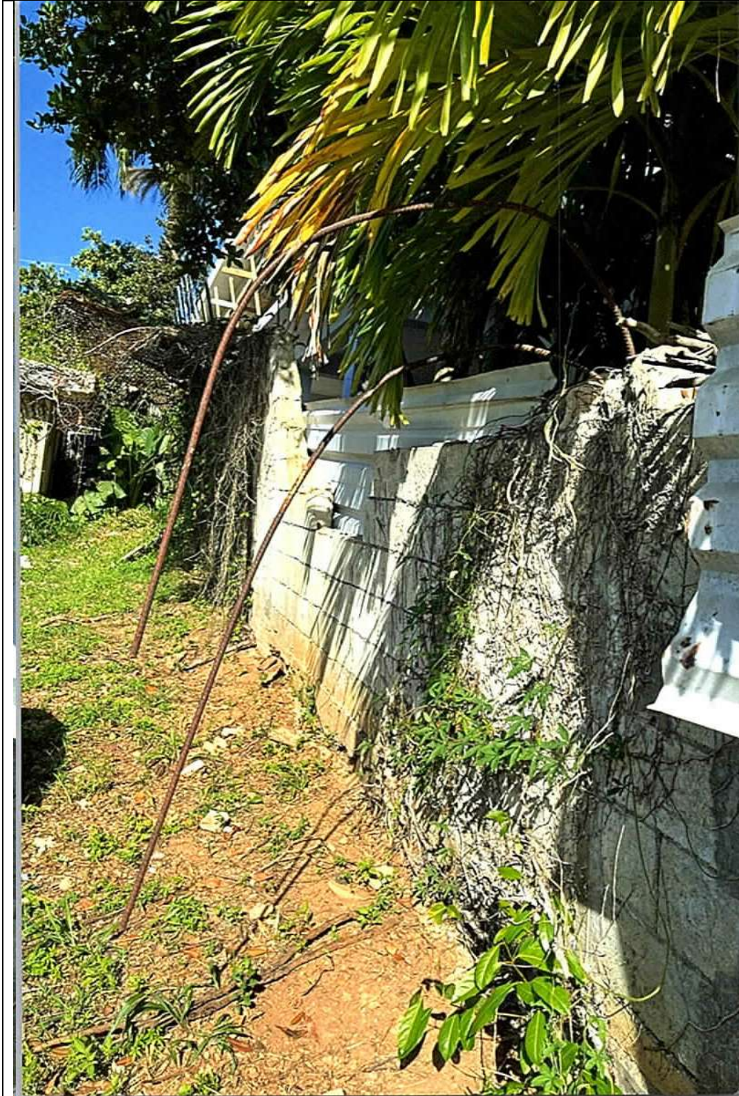
Photo No: 6 Location: South Retaining Wall
