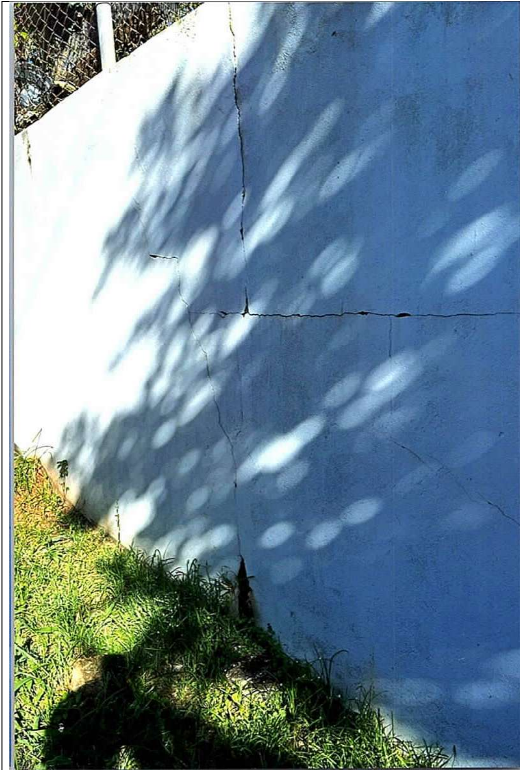
Photo No 2: Location: North retaining wall
