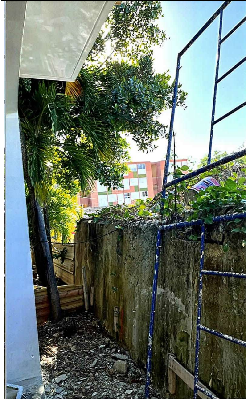
Photo No: 5 Location: South Retaining Wall
