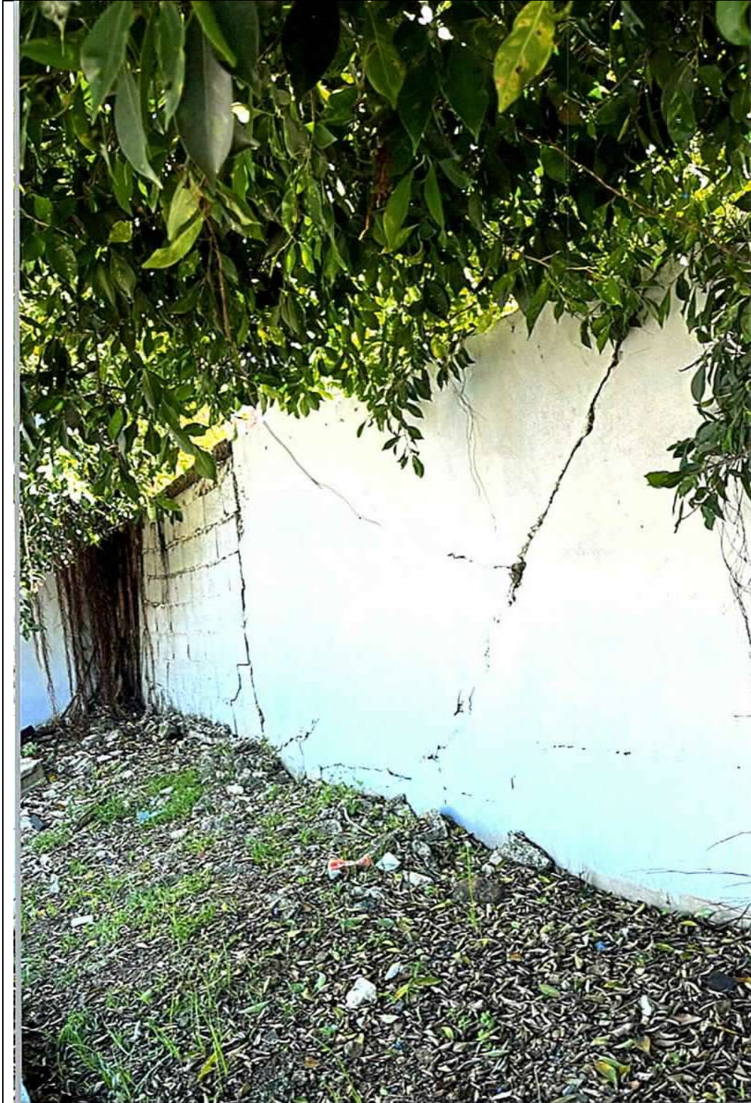
Photo No: 3 Location East retaining wall
