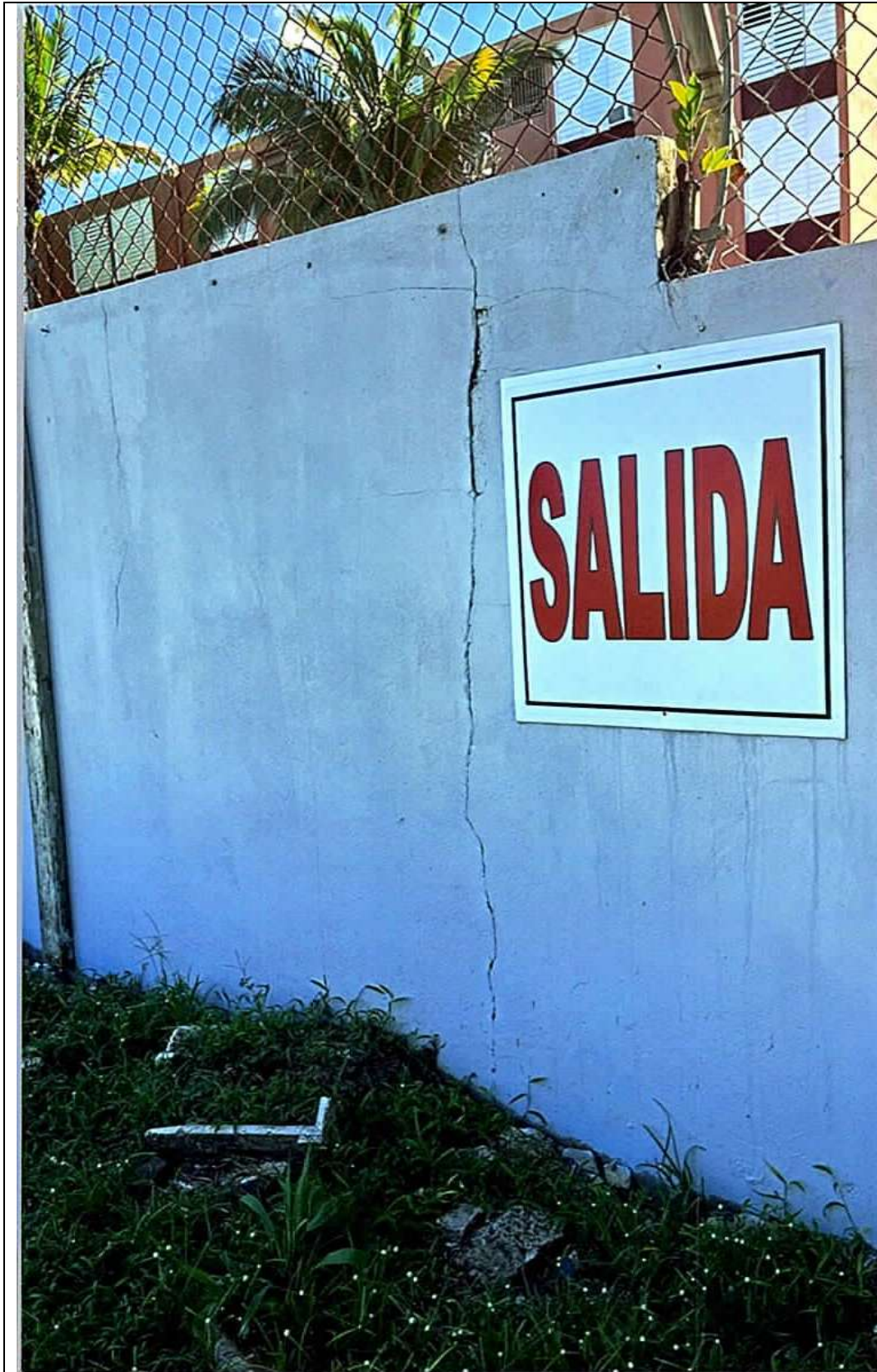
Photo No: 4 Location: East retaining wall
